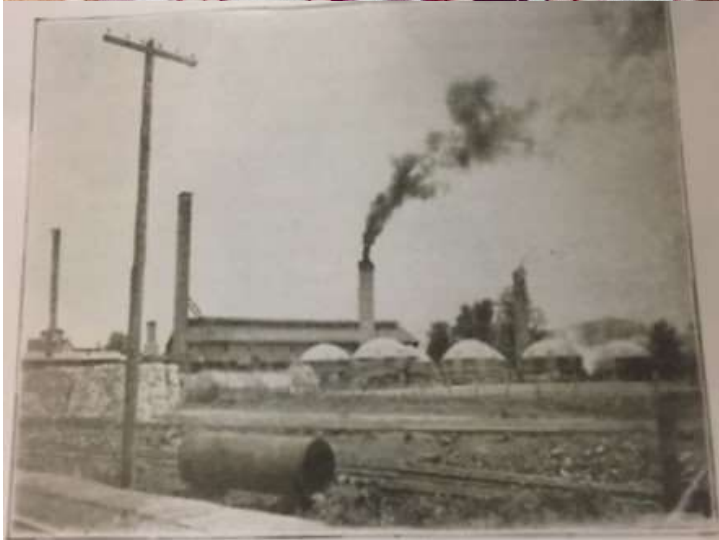
FIG. 33. Plant of the Davenport Brick and Paving Company, Buffalo, Iowa.
